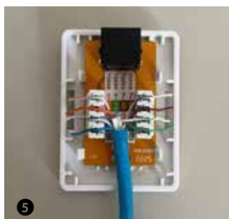
5 Push the wires into the IDC according to T568A/T568B color code
