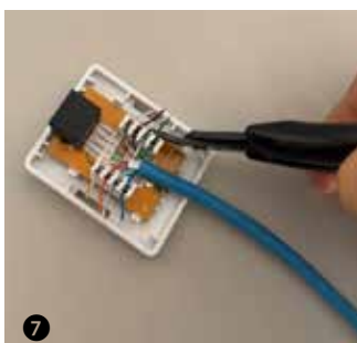
7 Trim the exposed wire cores
