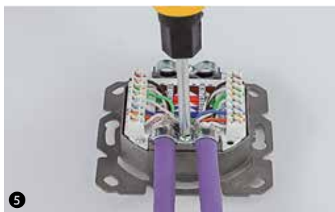
Tighten the shield clamp
