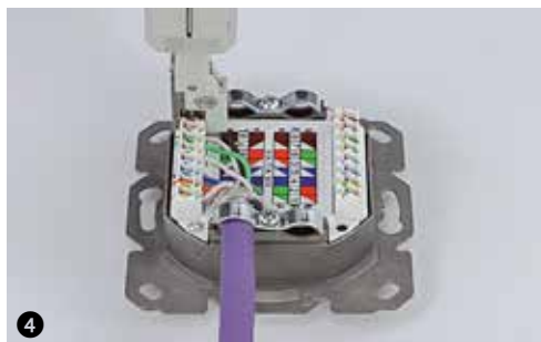
Terminate the wire pairs using an LSA tool
